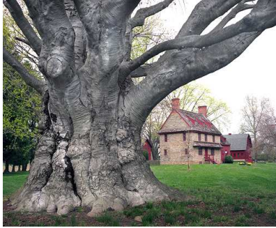
William Brinton 1704 House Photo by Fred Weyman, 2009
